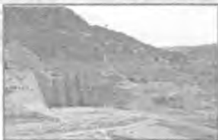
Re-construction of Bekhma Dam,
