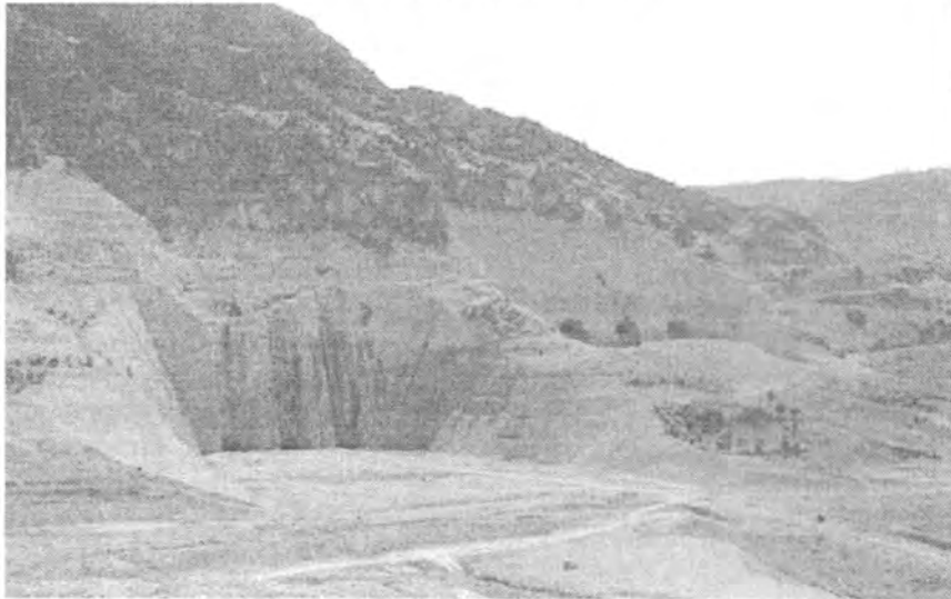
Intake Tunnels, fresh pictures
